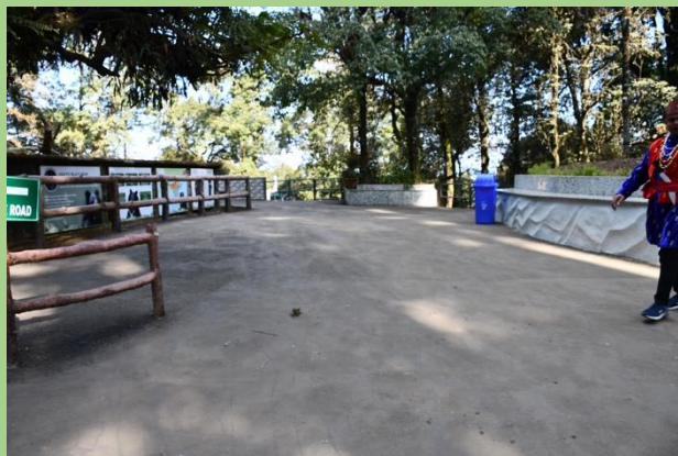
Fig: Renovation of bitumen road within the PNHZ Park
