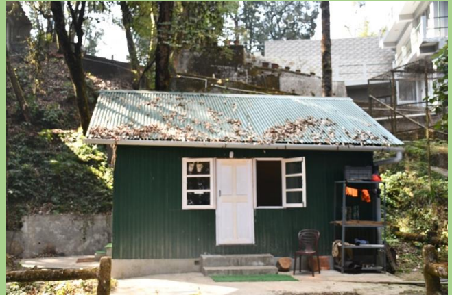
Fig: Construction of keepers house near veterinary hospital at PNHZ Park
